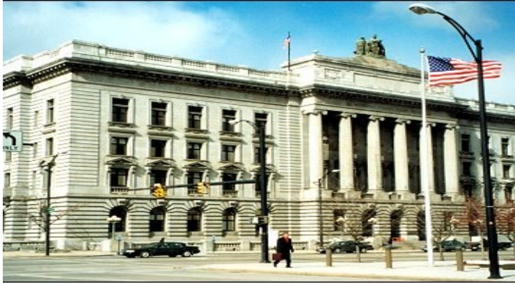
Mahoning County Court House
